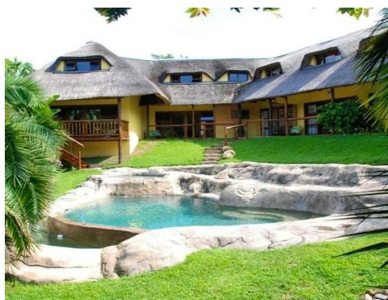
Sunny Rock Self Catering before renovations
