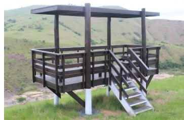
03 viewing platforms (decks) along the route were installed, 10m 2 each in size.
